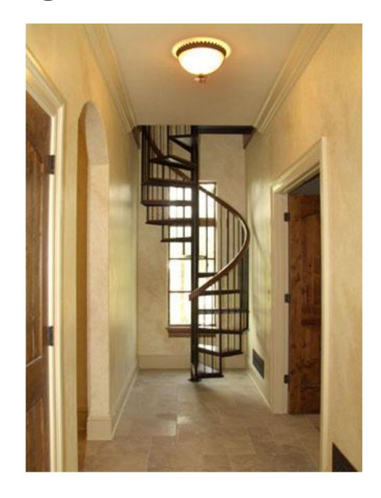
\*The minimum headroom for a flight of stairs is normally 6'-8". The exception to this is in the case of spiral stairs where the minimum headroom is 6'-6".
