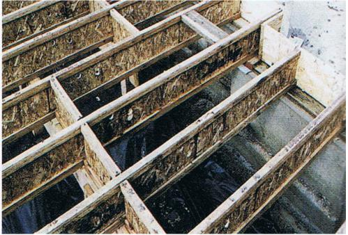
One component that is typically used when floor systems such as a concrete slab and a floor joist system are combined is the ledger. It is used to support the floor joists and sub-floor when they intersect the concrete.
