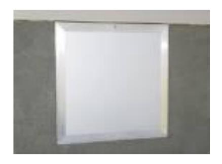
If the crawl space access is located in the floor it should be at least 18 inches by 24 inches. If it is located in the foundation wall it can by 16 inches by 24 inches.
