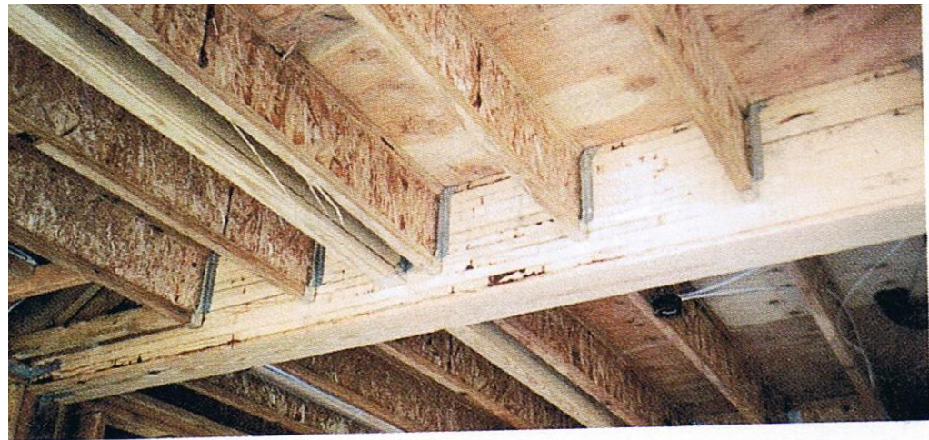
FIGURE 25.5 ■ A western platform floor system constructed using
